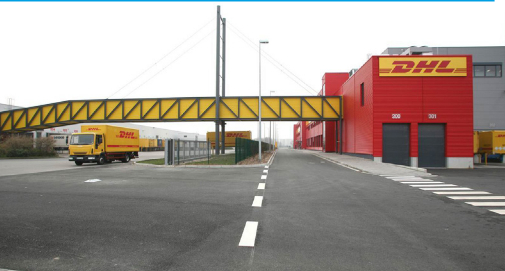
Exterior view of the DHL logistics centre in Greven, Germany.
